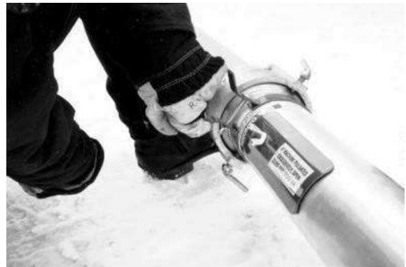
Fig. 4-5 Intake Installation
