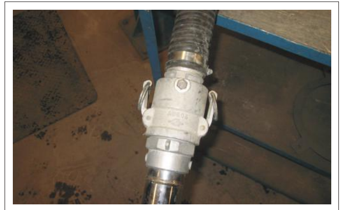
FIG. 25 COUPLER (TYPICAL)
