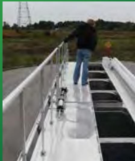
*Air operated hand rail on the catwalk.*
