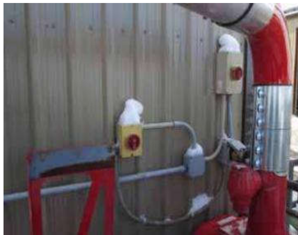
Figure 12 - Power Disconnect
