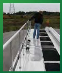
Air operated hand rail on the catwalk.
