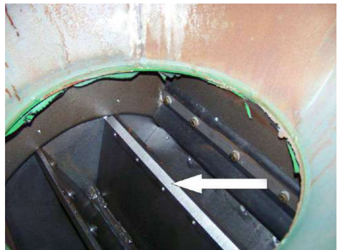
Fig. 5-27 Checking Tip Clearance Through The Access Door.
